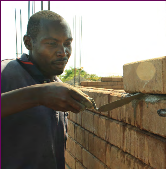
Roche villager laying ISSB bricks for Roche Health Center
